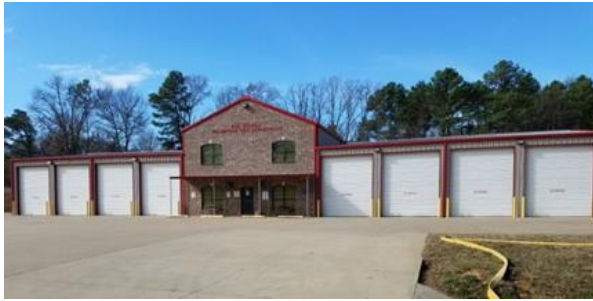
Figure 130: Red Springs VFD, Station 1
